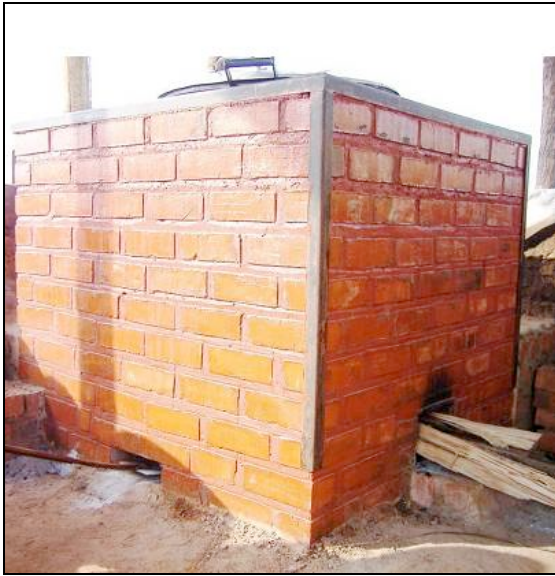
Figure 7. Institutional rocket stove made with bricks 7
